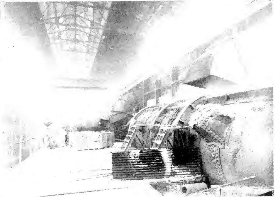
Fig. 72—Interior of Converter Building, Canadian Copper Company, Copper Cliff, Ontario.
